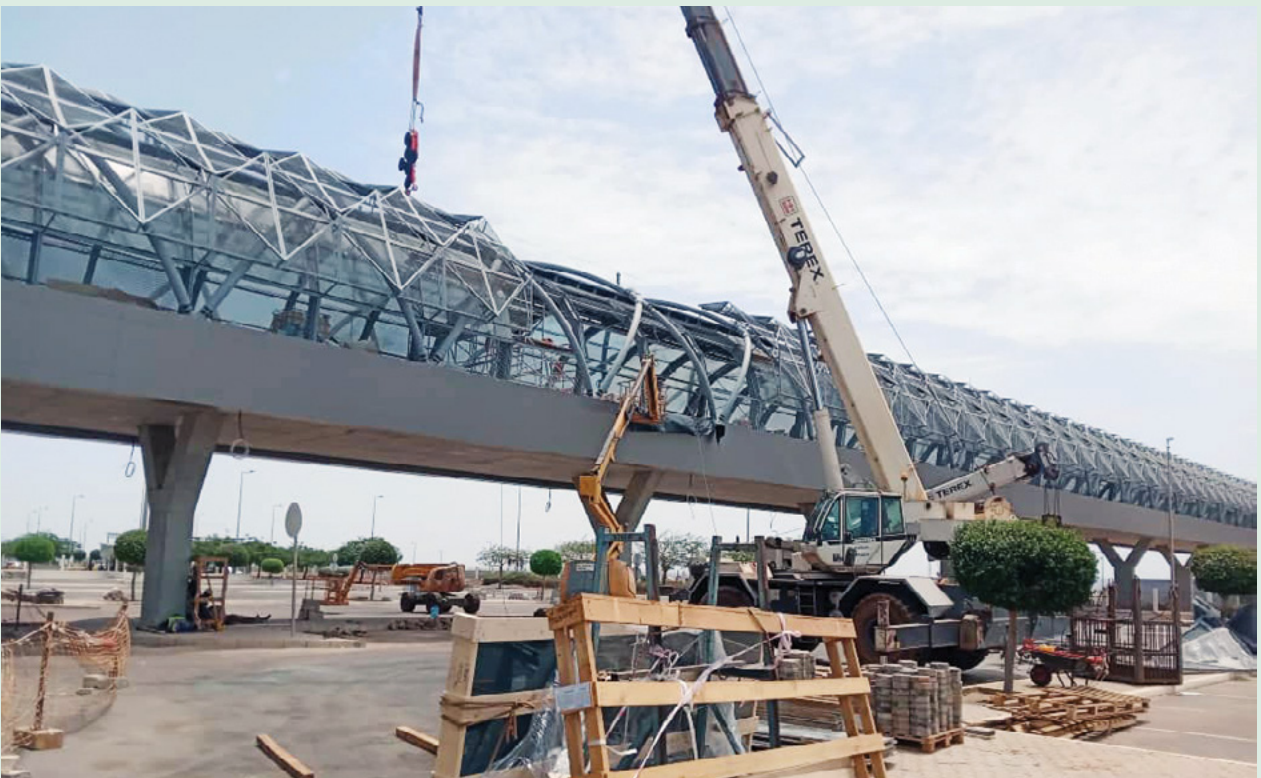
TER-Airport Bridge, Senegal
